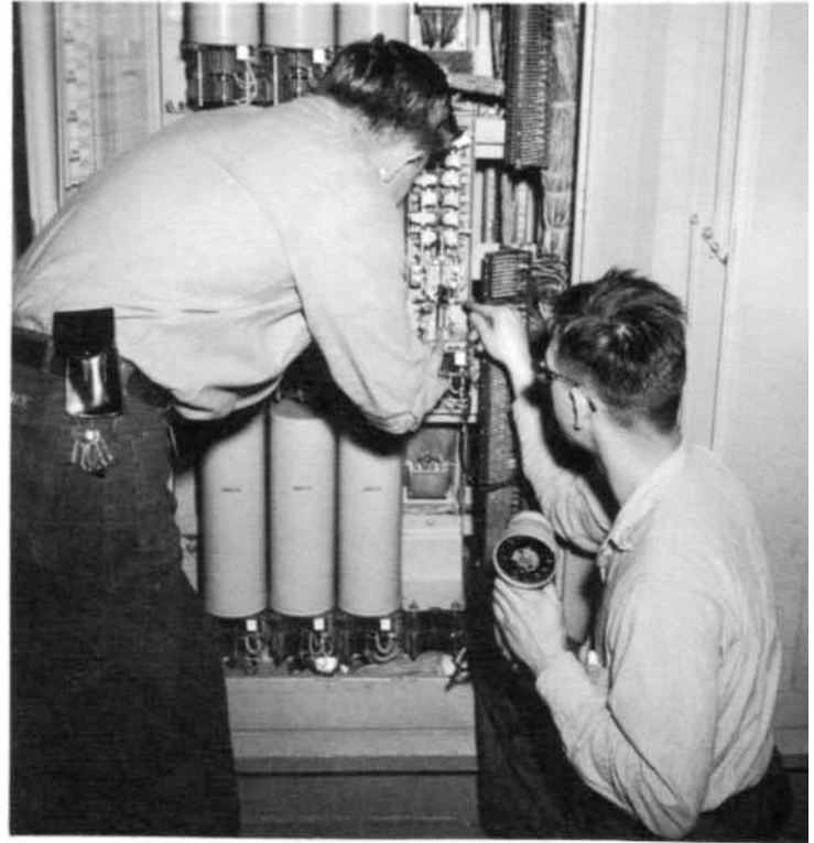
... IC Electricians Page and Naylor check out telephone circuits
